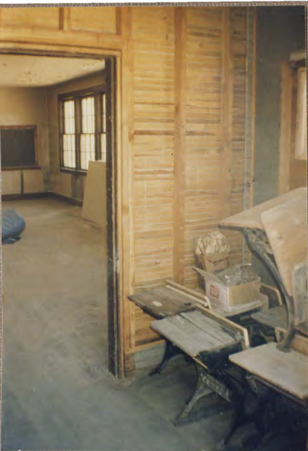
Ready For New Wall
