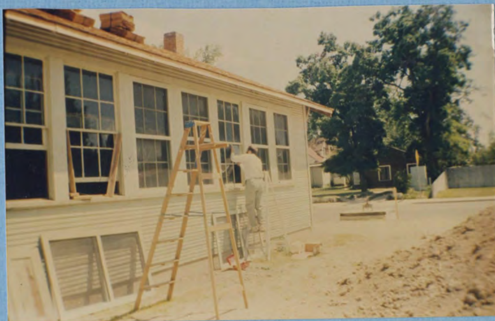
REV. KENT ROBERTS Repairs Windows
