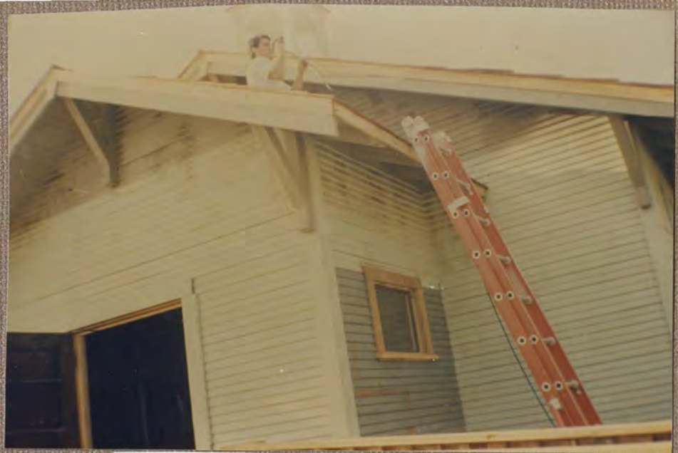
Installing Power For Flagpole Light
