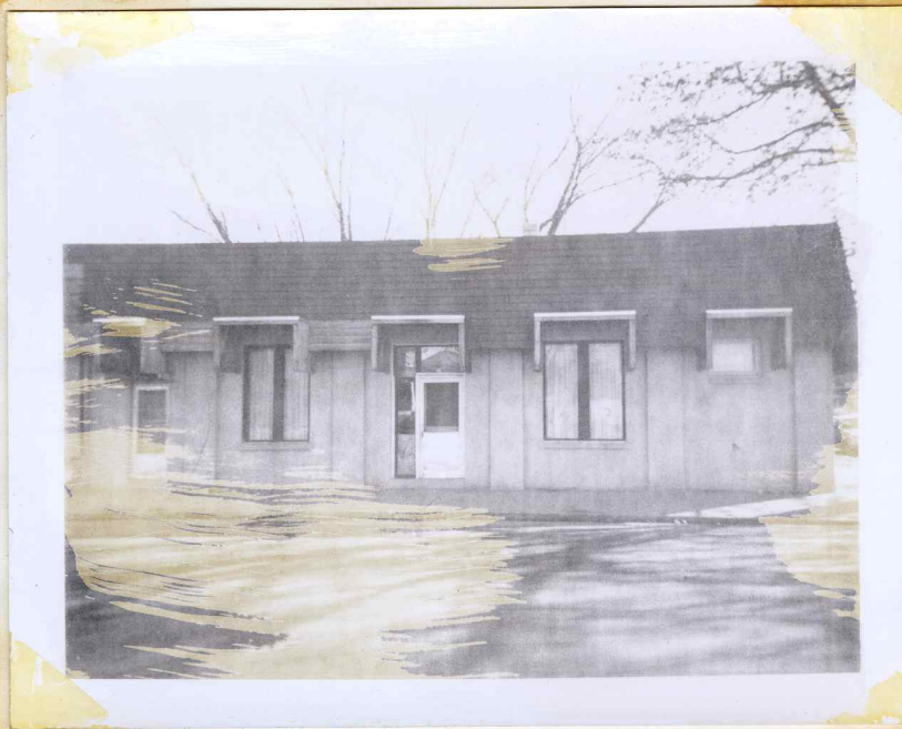
Occident Club Room in which the Emergency Loan Closet is housed.
